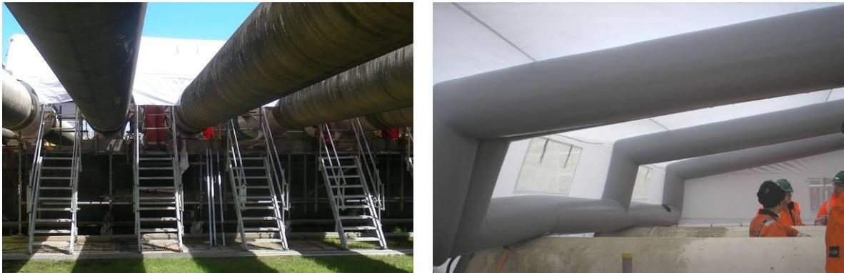
Figure 10. Smart access options: movable scaffolding on rails (after removal of stairs) and inflatable weather protection.
